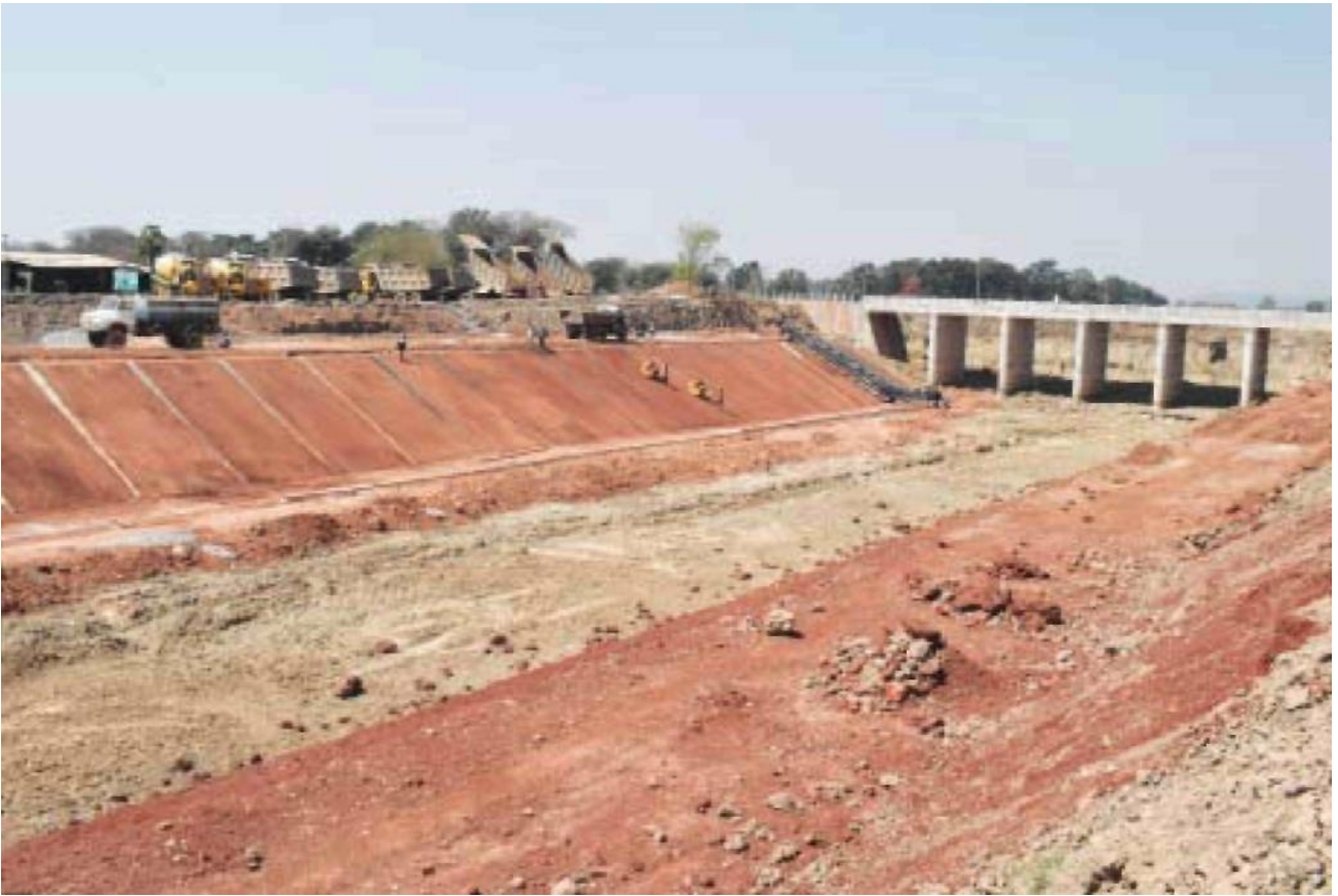
Lining work in progress (Baitarani Left Bank Canal of Anandapur Barrage)
