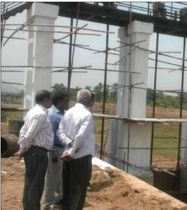
Roof slab casting of Rengali Irrigation Project
