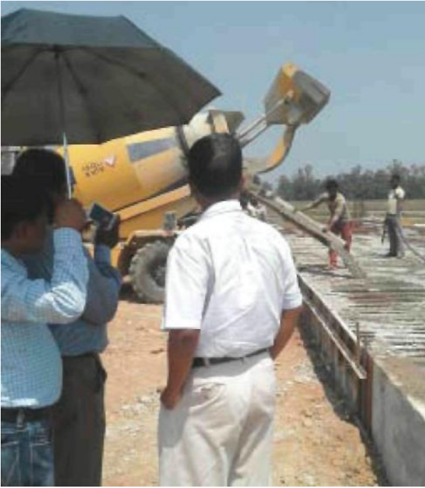
Slab Casting of CD 57 of Kanpur Canal
