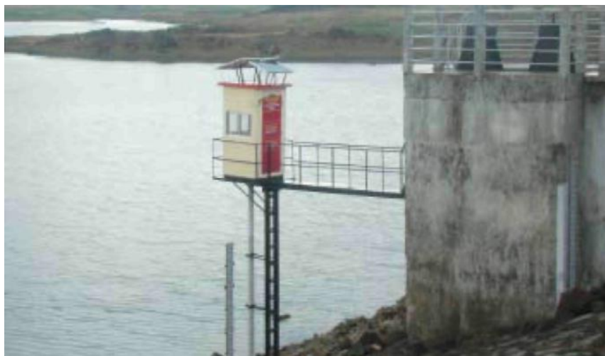
Installation of Automatic Water Level Recorder at Nesa Dam
