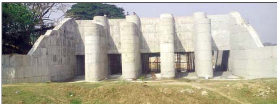
Sluice constructed at Baranga under RIDF (Mirichia-Jhirkidia Gherry)
