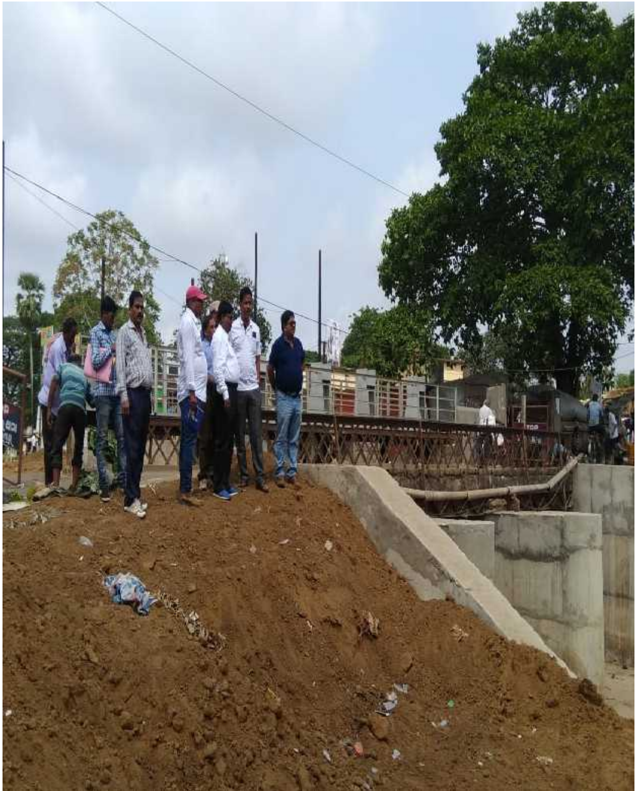
Balichandrapur CR-cum-Fall at RD. 36.85
