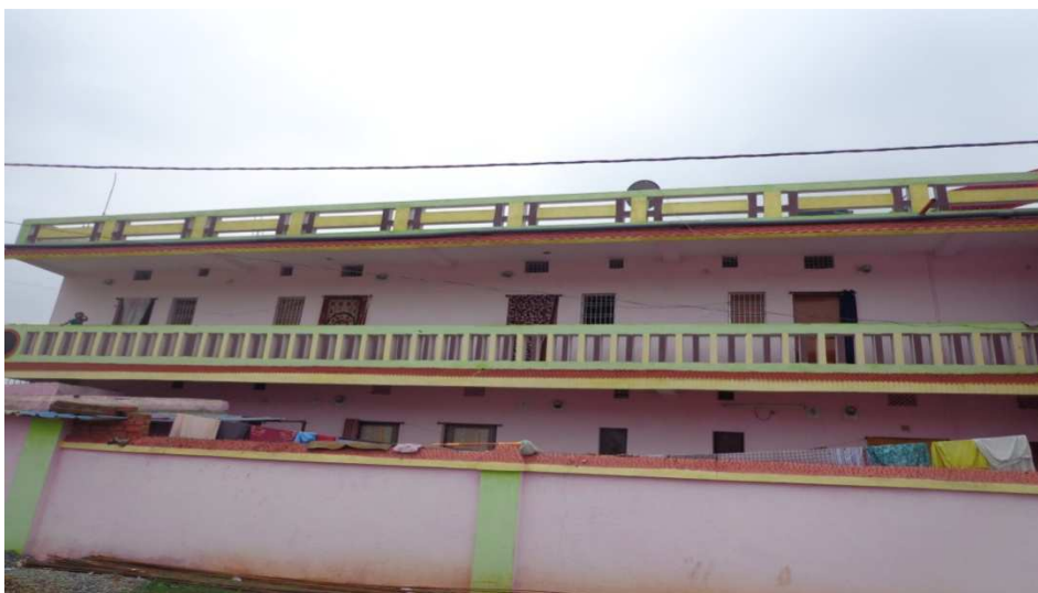
3- House of Sri Hemsagar Patel, Ekatali, Jharsuguda where Private RRHS structure is installed.
