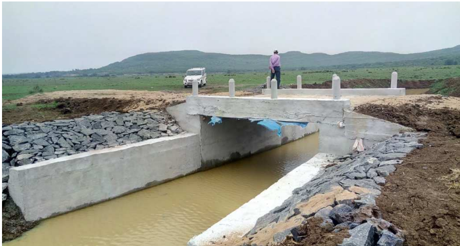
Foot Bridge over Link Drain of Sapua Nalla in Athagarh Area.
