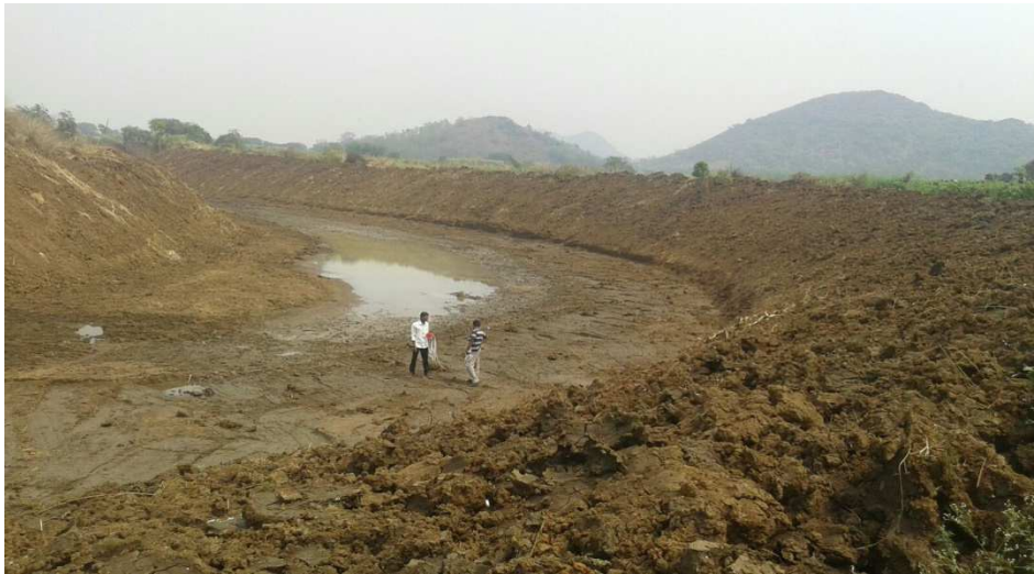
Renovation Works of Kaligiri Nalla in Progress( Banki)
