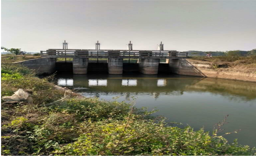
Check Dam on Telijore Nalla (Banambarbandha) of Kantapada Block.
