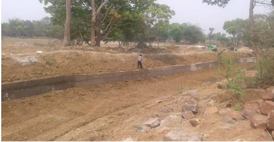
Slope Protection Works in Krishnapalli Link Drain (Banki)
