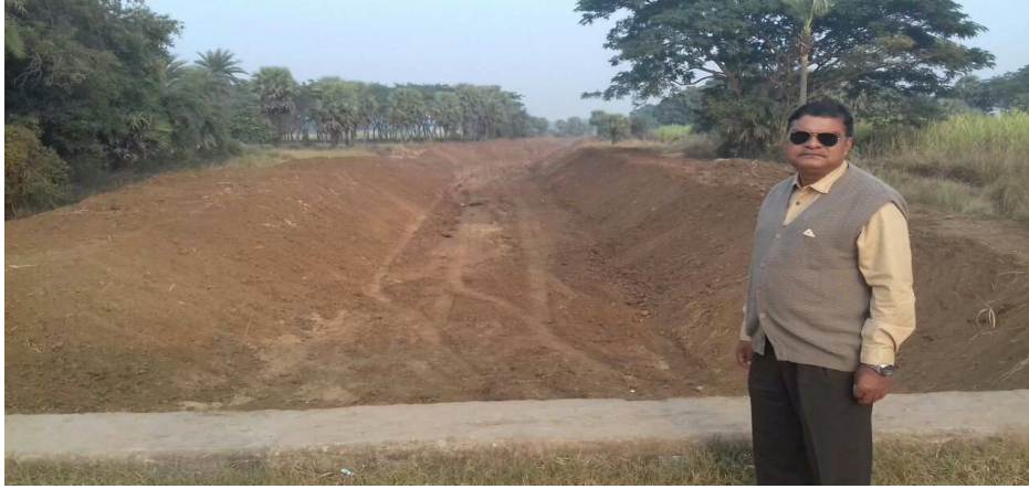
Renovation Works of Malia Drainage System in Progress (Bailish Mouza)
