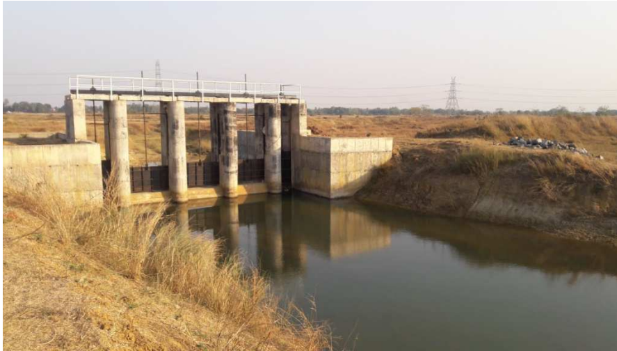
Check dam over GandhaNadi near Panchamania at RD 17200 m. in Athagarh.
