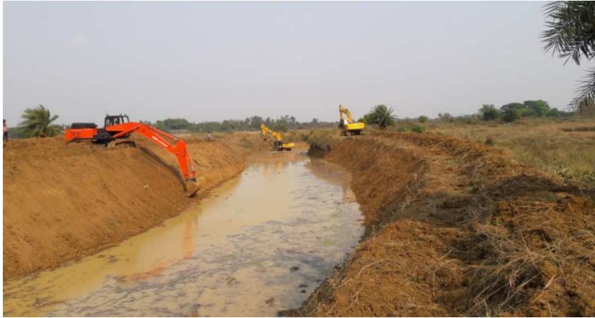
Renovation Works of Gandha nadi in Progress.
