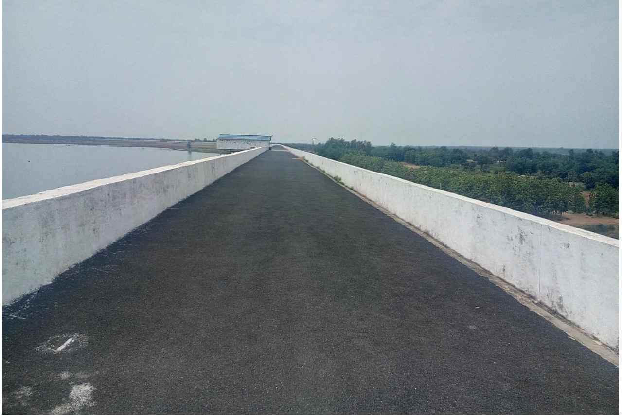
JAMBHIRA EARTH DAM TOP BANK ROAD AND PARAPET WALL
