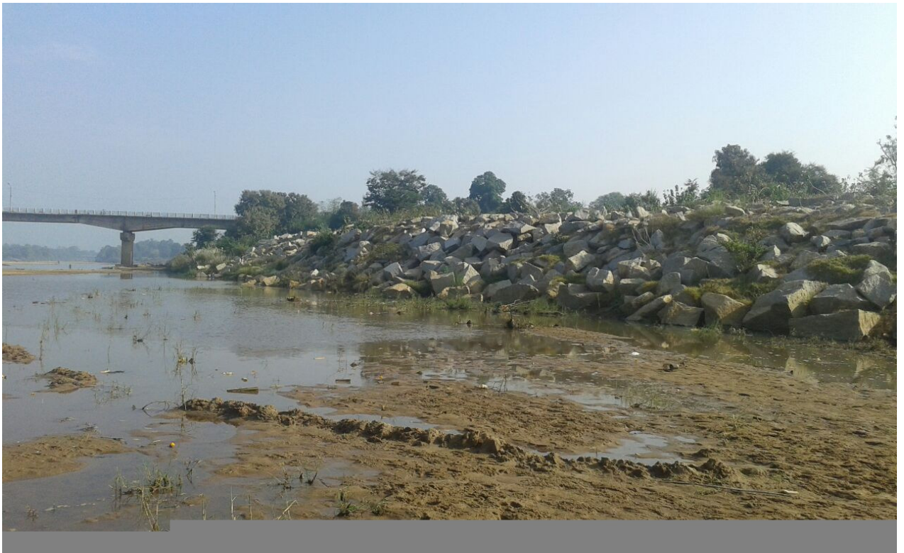
Launching apron at Gudari under NABARD Assistance vide Agreement no. 58-P1/2015-16 (work in progress)
