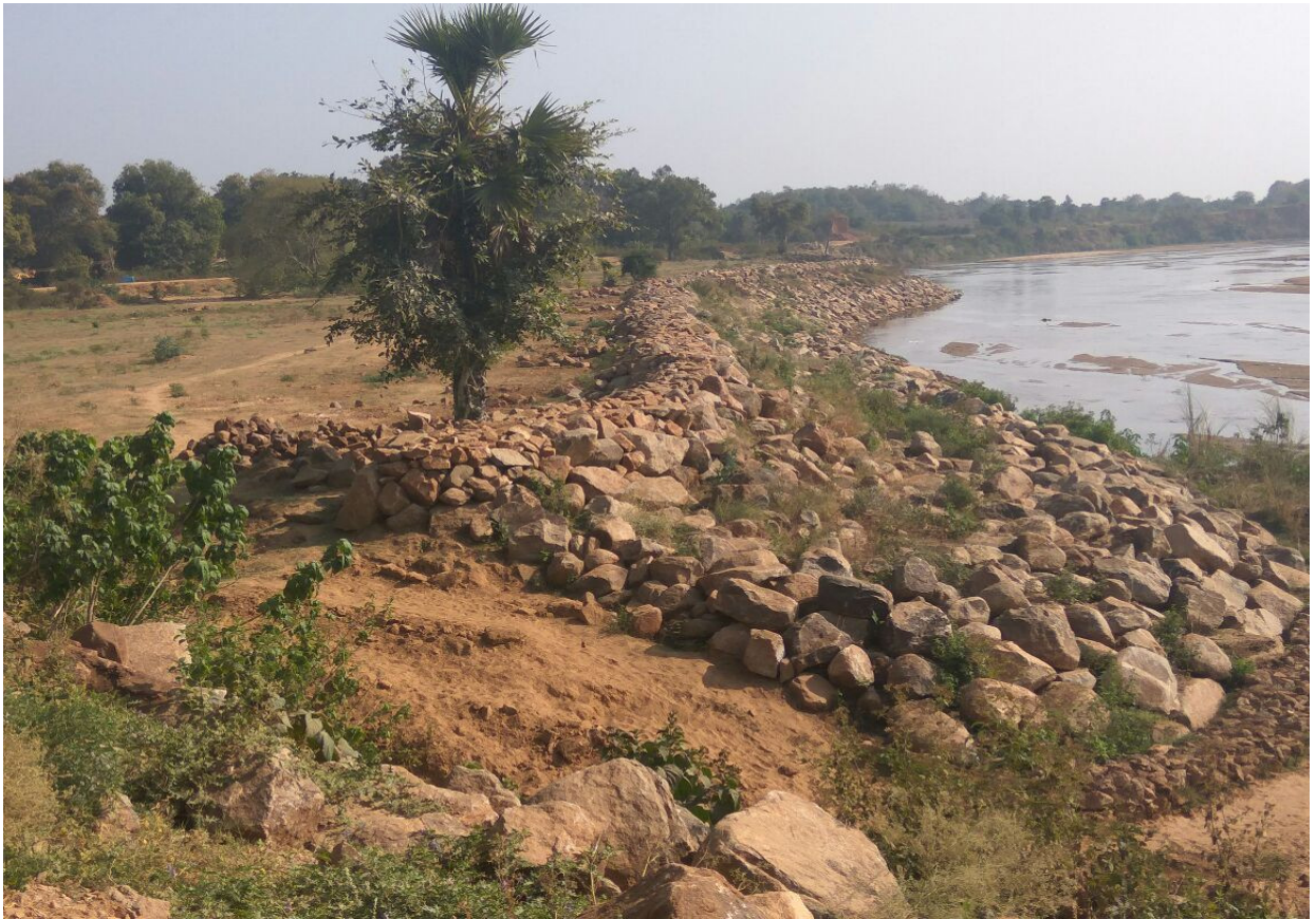
Launching apron at Gudari under NABARD Assistance vide Agreement no. 58-P1/2015-16 (work in progress)
